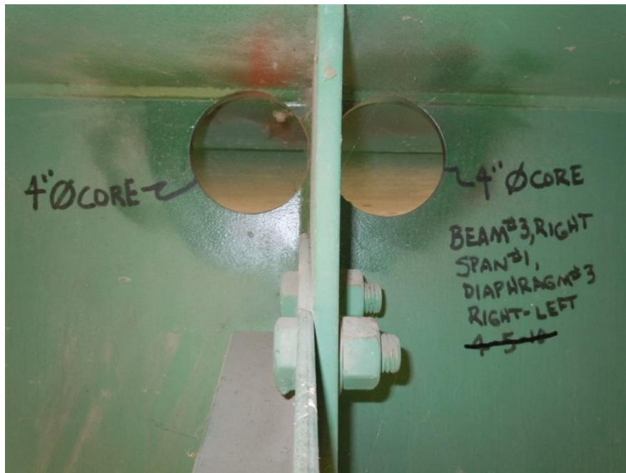
Figure 6.2.10-1. Diaphragm Connection Stiffener Fatigue Crack Retrofit
