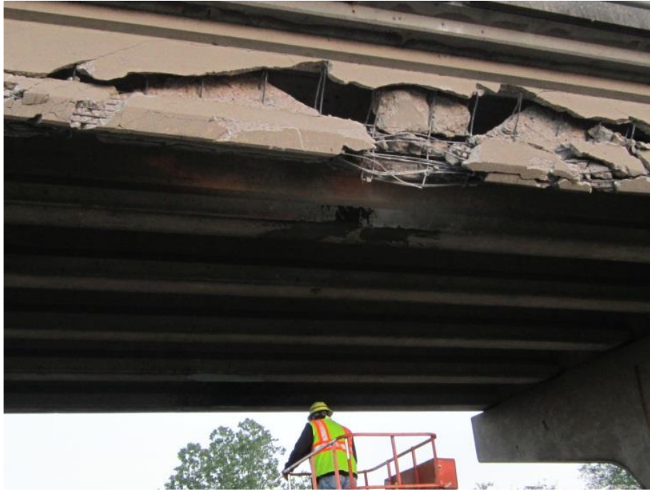
Figure 2.9.3.2-6. Severe Prestressed Beam Damage with Excessive Concrete Section Loss
