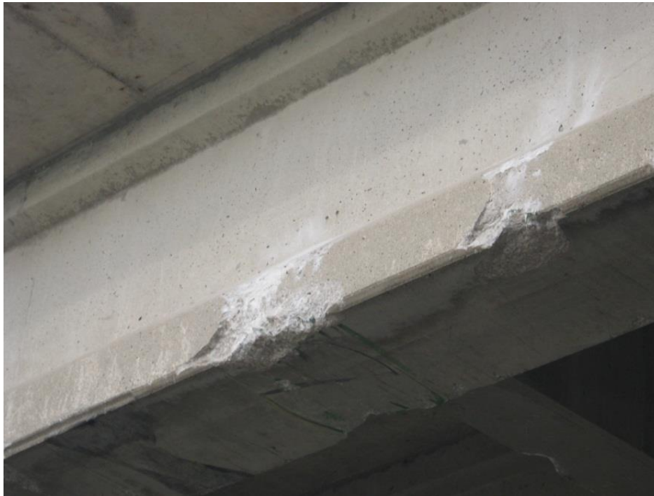
Figure 2.9.3.2-2. Minor Bottom Flange Spalling
