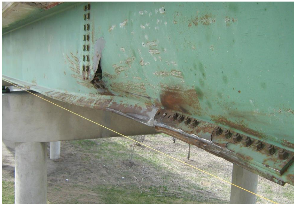
Figure 2.9.3.1-4. Out of Plane Bending with Web Tear
