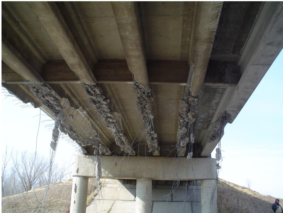
Figure 2.9.3.2-7. Multiple Prestressed Beams with Severe Damage
