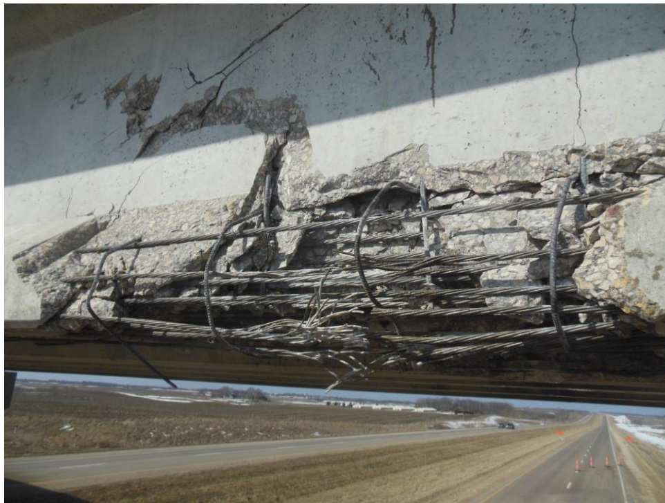
Figure 2.9.3.2-5. Heavy Damage with Web Cracking and Severed Mild Reinforcing and Prestressing Strands
