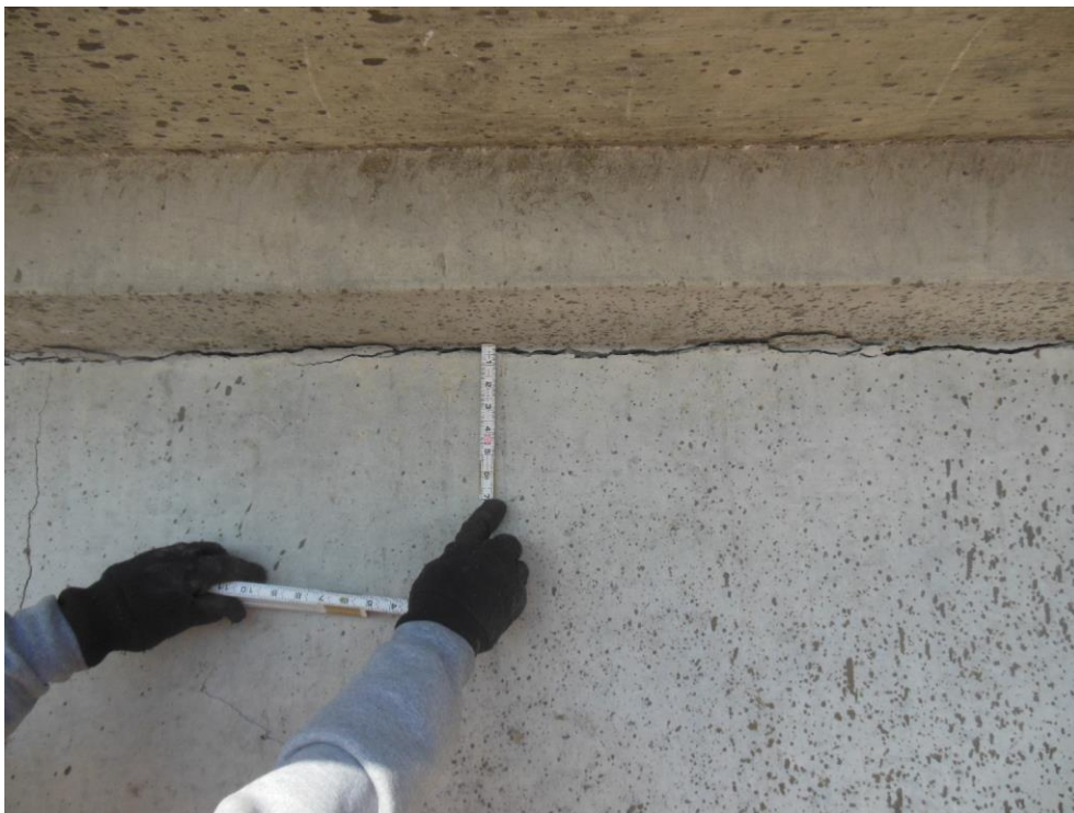
Figure 2.9.3.2-4. Cracking Along Web-to-Top Flange Interface
