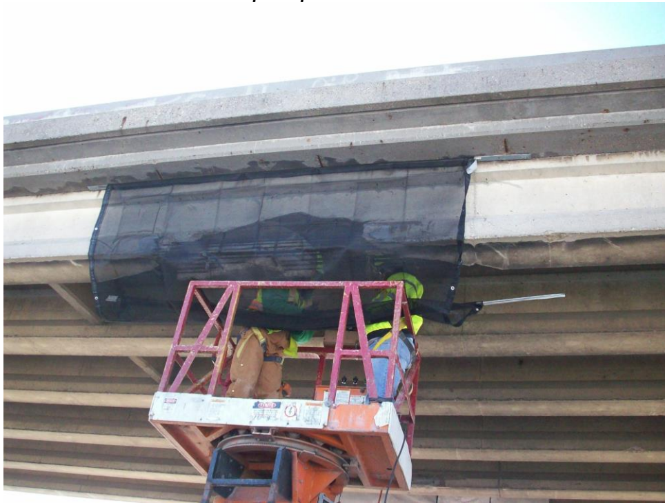
Figure 2.9.3.2-1. Installation of Drape to Catch Loose Debris
