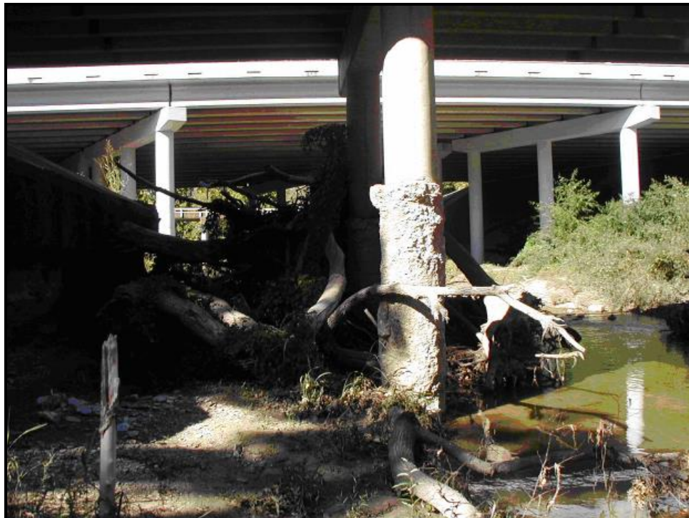
Figure 5.1.4. Bridge Pier Scour Damage
