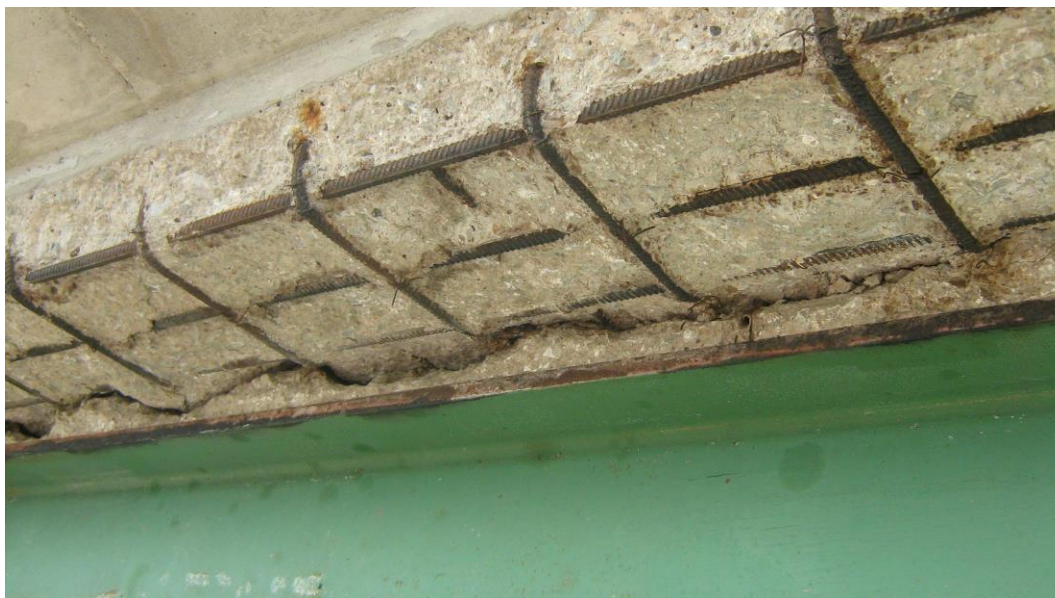
Figure 2.9.3.1-5. Bottom of Deck Spalling with Crack at Girder-to-Deck Interface
