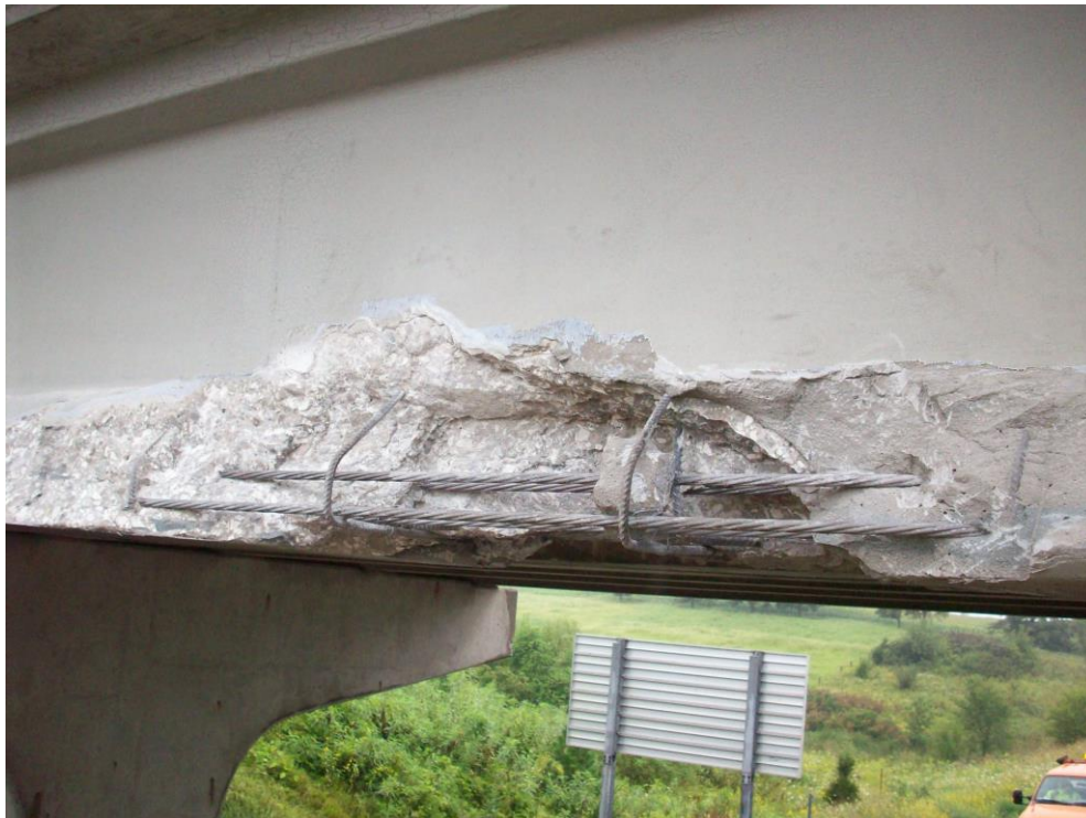
Figure 2.9.3.2-3. Bottom Flange Damage with Mild Reinforcing and Prestressing Strands Intact
