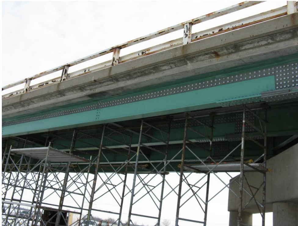
Figure 3.2. Partial Steel Beam Removal and Replacement
