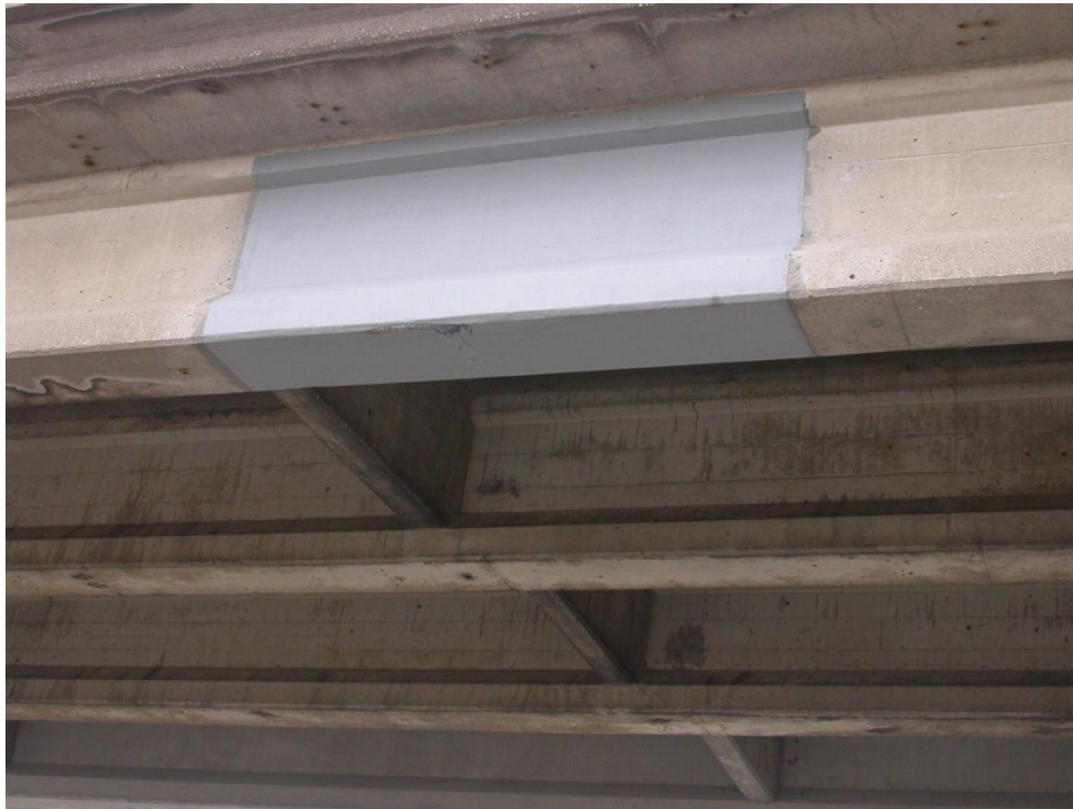
Figure 4.2. Fiber Reinforced Polymer Wrapped Repair
