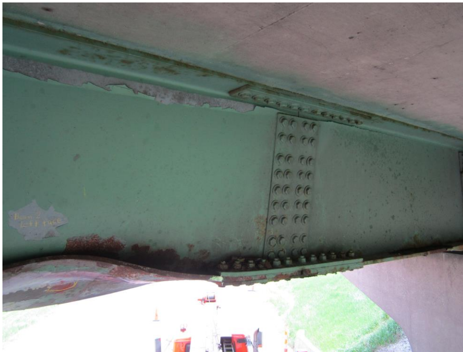
Figure 2.9.3.1-2. Moderately Bent Bottom Flange with Some Web Distortion
