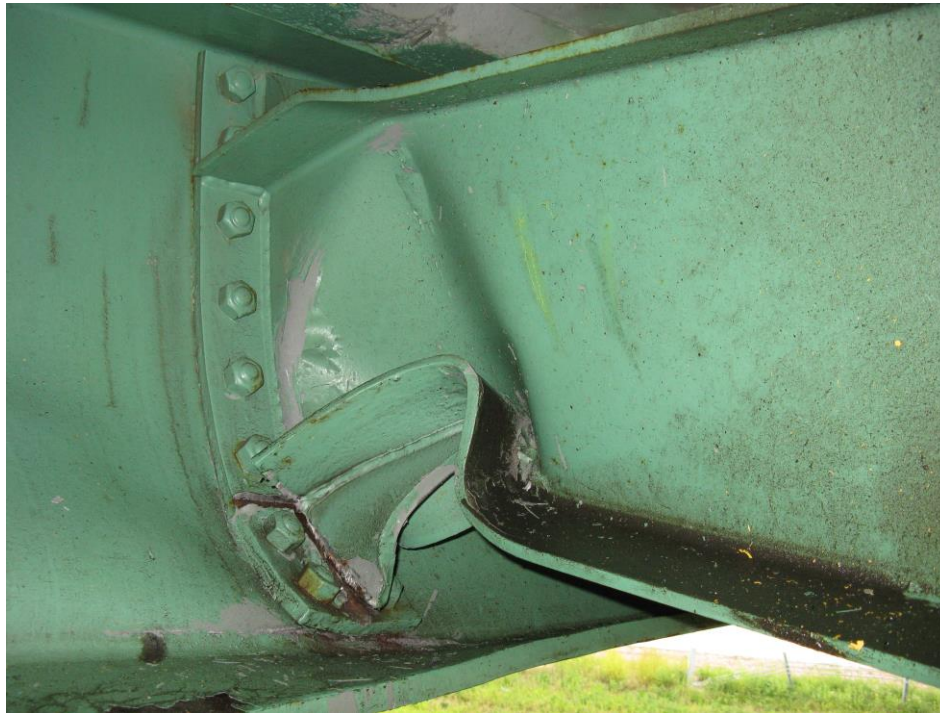
Figure 2.9.3.1-3. Damaged Diaphragm Member
