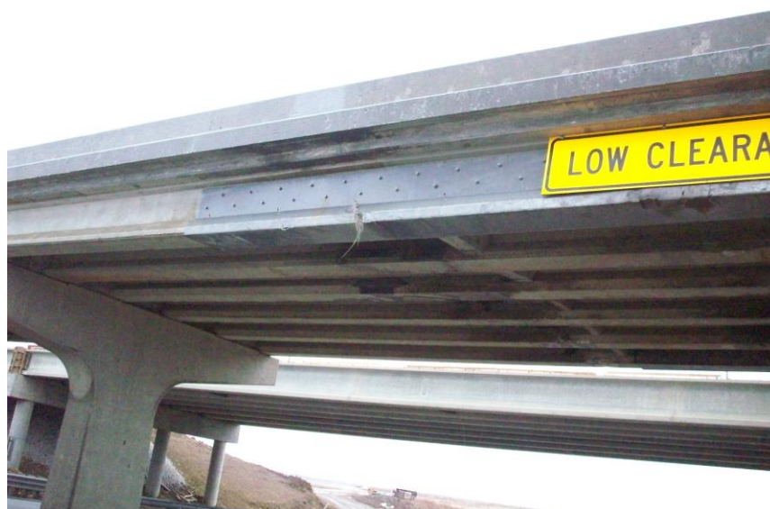
Figure 4.3. Grouted Steel Sleeve Repair
