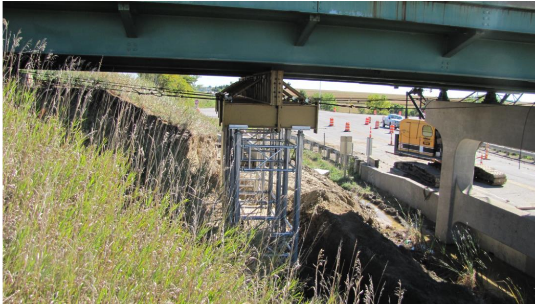
Figure 3.4-2. Shoring Tower Providing End Span Support
