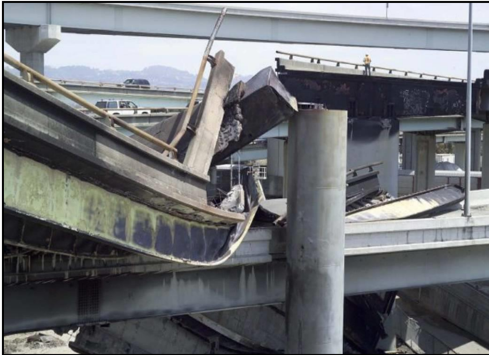
Figure 5.1.1. Collapse of I-880 Bridge in San Francisco from Fire Damage
