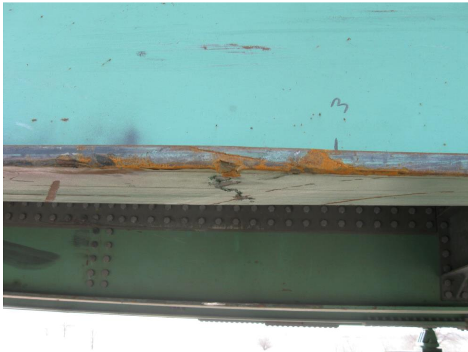
Figure 2.9.3.1-1. Steel Gouge and Paint Scrape
